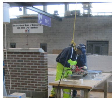
7/4" Circular Saw with water drip from hose cutting stone
